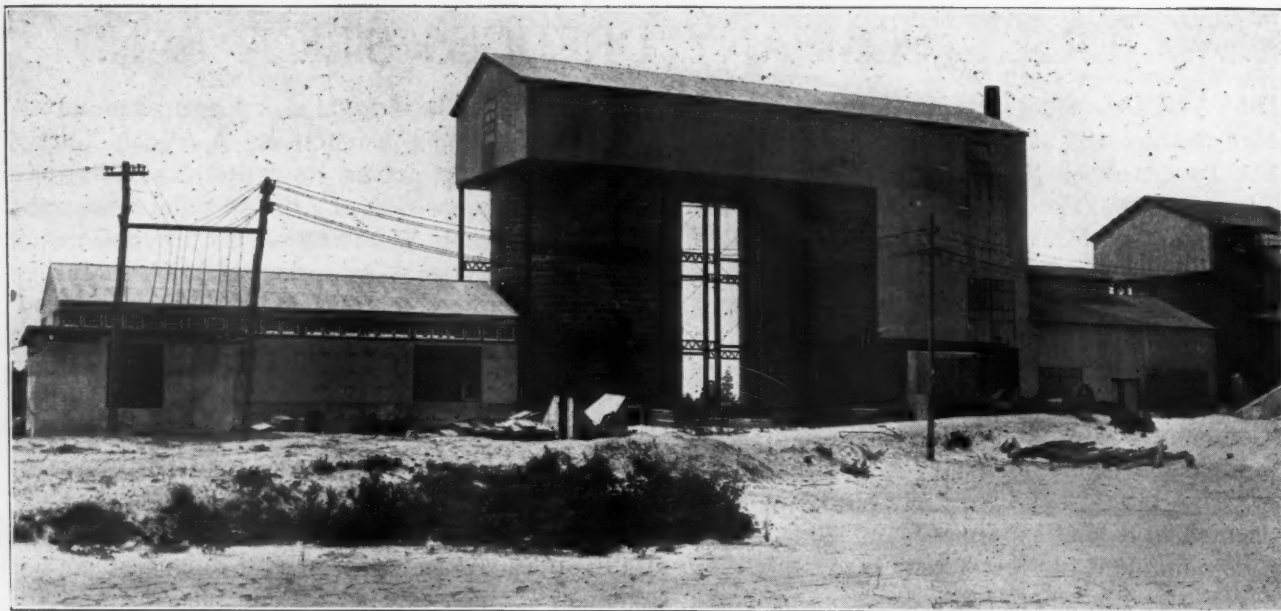
The Two Hollow Clay Tile Storage Bins for Final Storage
